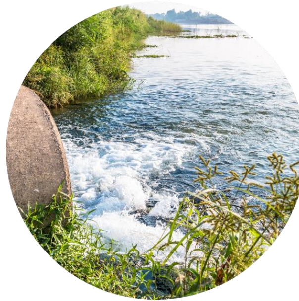
Urban sewage, CSU Colorado Water Quality
